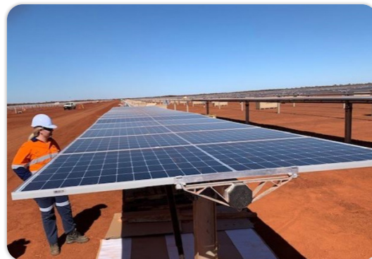
Pictured – First solar panels being installed at Chichester solar farm.
