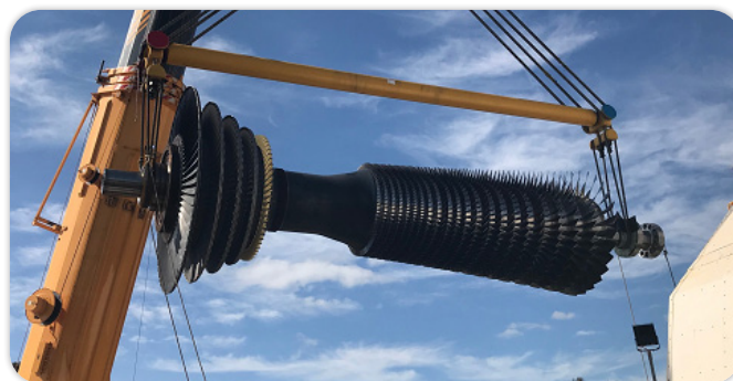
Pictured – Wagerup turbine upgrades in progress.
