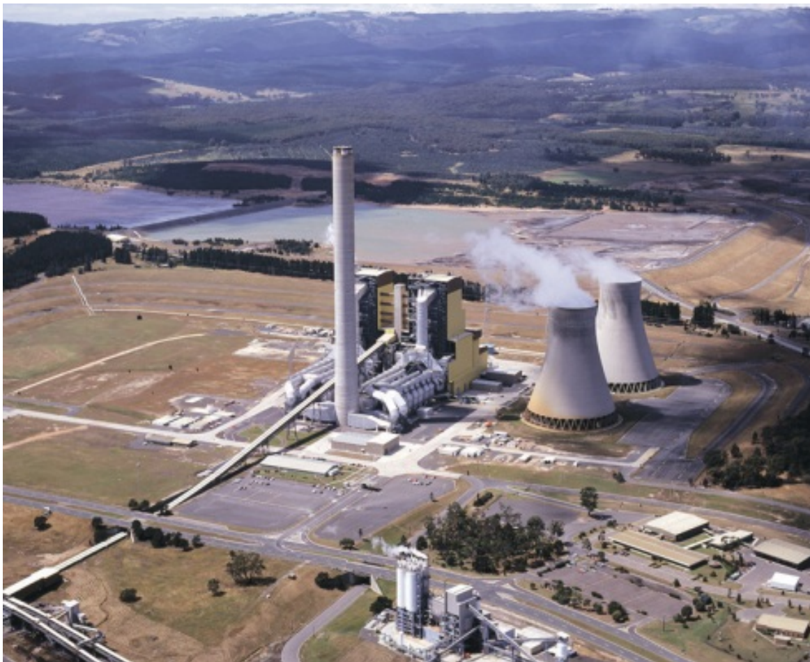
Figure 1- Aerial of Loy Yang B Power Station. Ash holding dams in the background.
